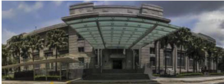
Family and Juvenile Court building in 2013, after the restoration works
